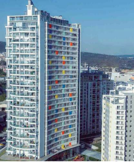
SURYAPI / MIRAGE PROJESİ
